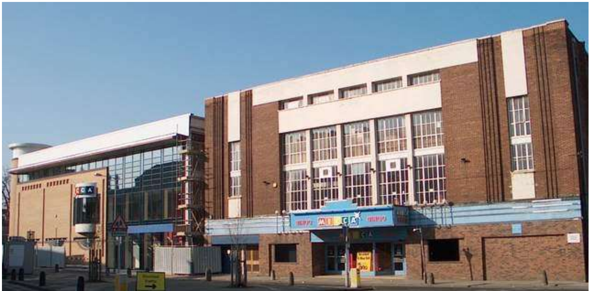
The Rialto shortly before demolition in 2003. The MECCA bingo hall had just been built on the corner of Blue Bridge Lane, ready to take over from the former cinema
