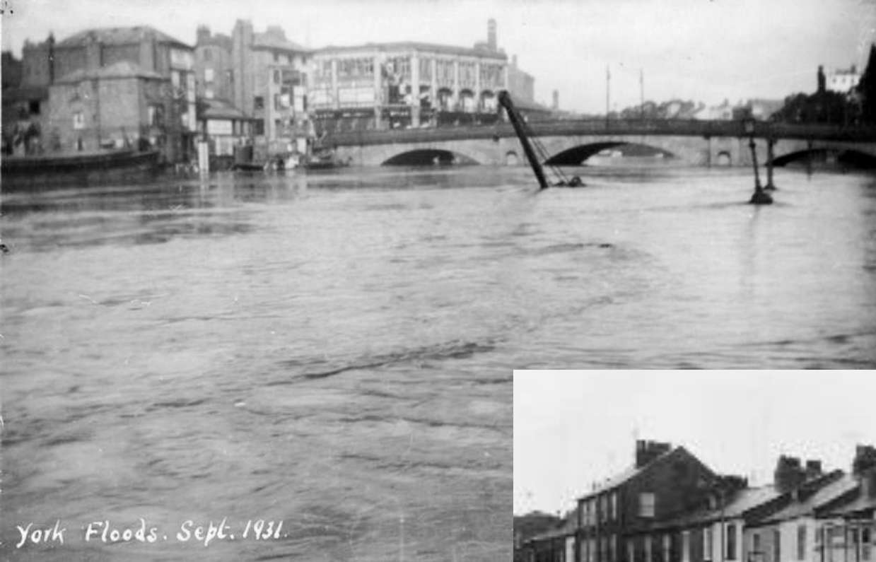
Flooding at King's Staithe 1931
