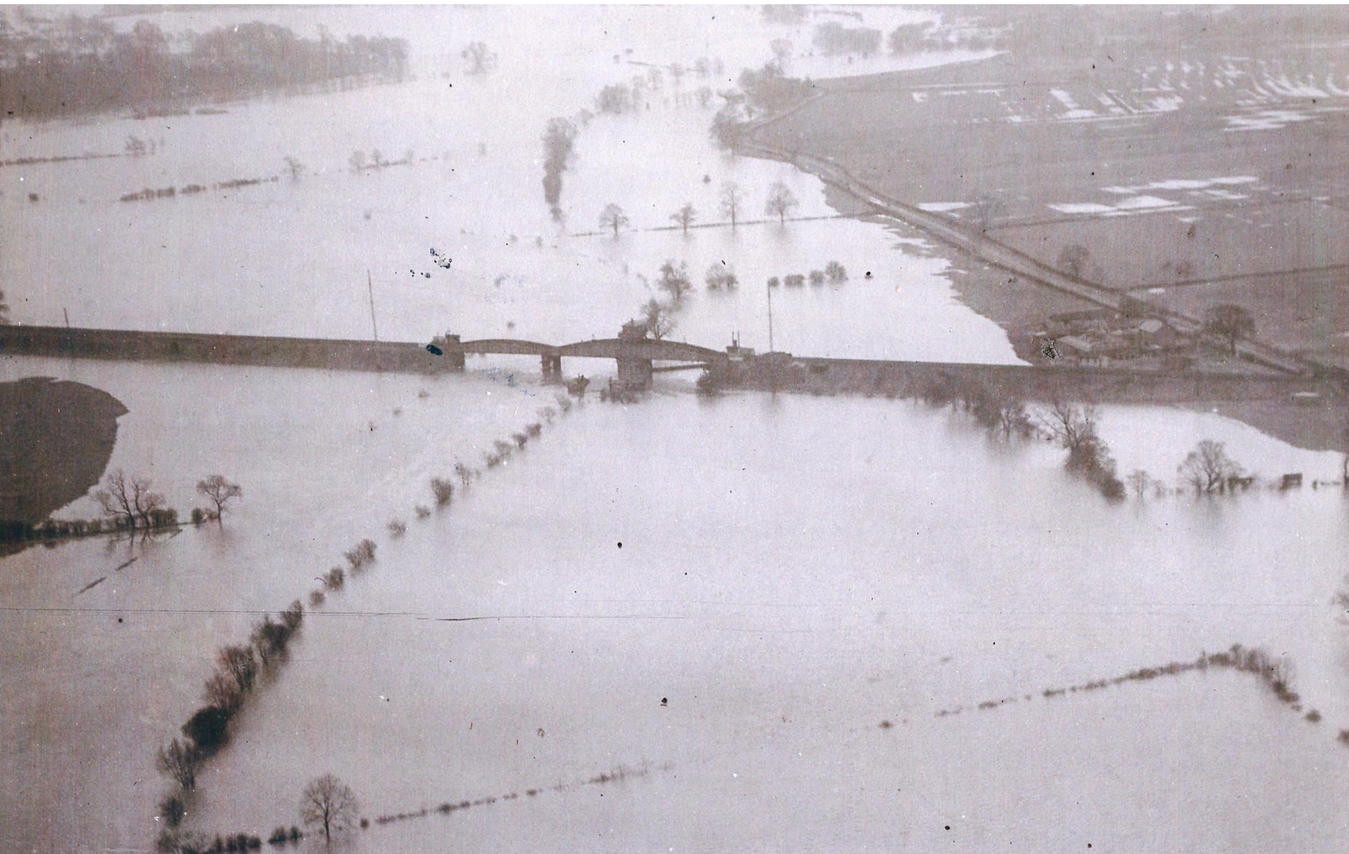
Naburn Swing Bridge 1947
