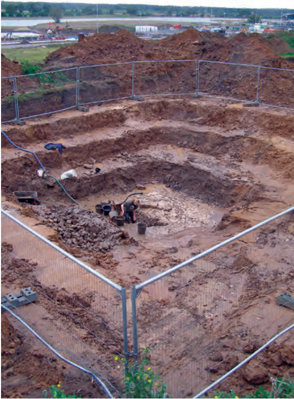
The challenge of excavating a deep well
