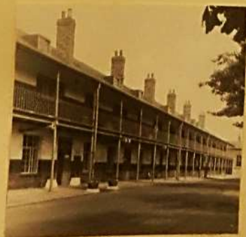
VIEW FROM TETHERING GREEN BALCONY ADDED 1862.
