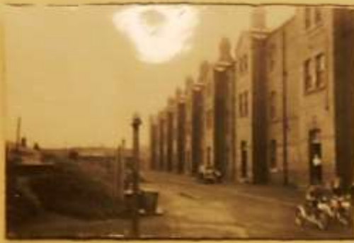
VIEW OF MAIN ENTRANCE FACING BOUNDARY WALL.
