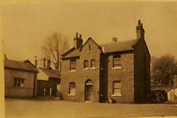
VIEW OF BLOCK IN CAVALRY BARRACKS
