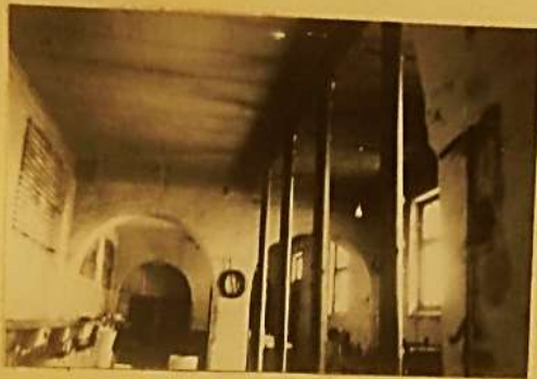
INTERIOR OF STABLES SHOWING FILLER JOIST FLOOR.
