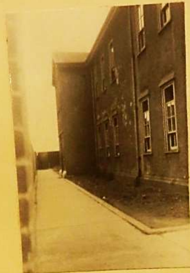
'LIGHT CONSTRUCTION'. BARRACK BLOCK.
