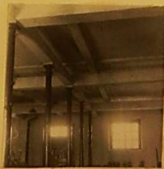
INTERIOR OF STABLES SHOWING TIMBER FLOOR.
