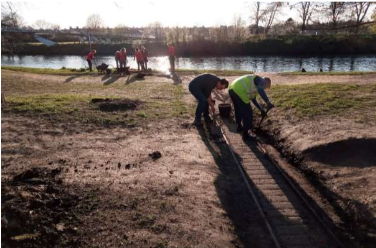
Goodgym volunteers digging out the tracks at the Ordnance Depot wharf
