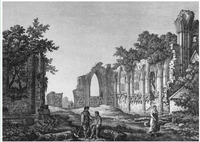
Above: St Mary's Abbey, Joseph Halfpenny, 1807. Engraving of the view from the south-east showing the inner sides of the north and west walls of the nave.
