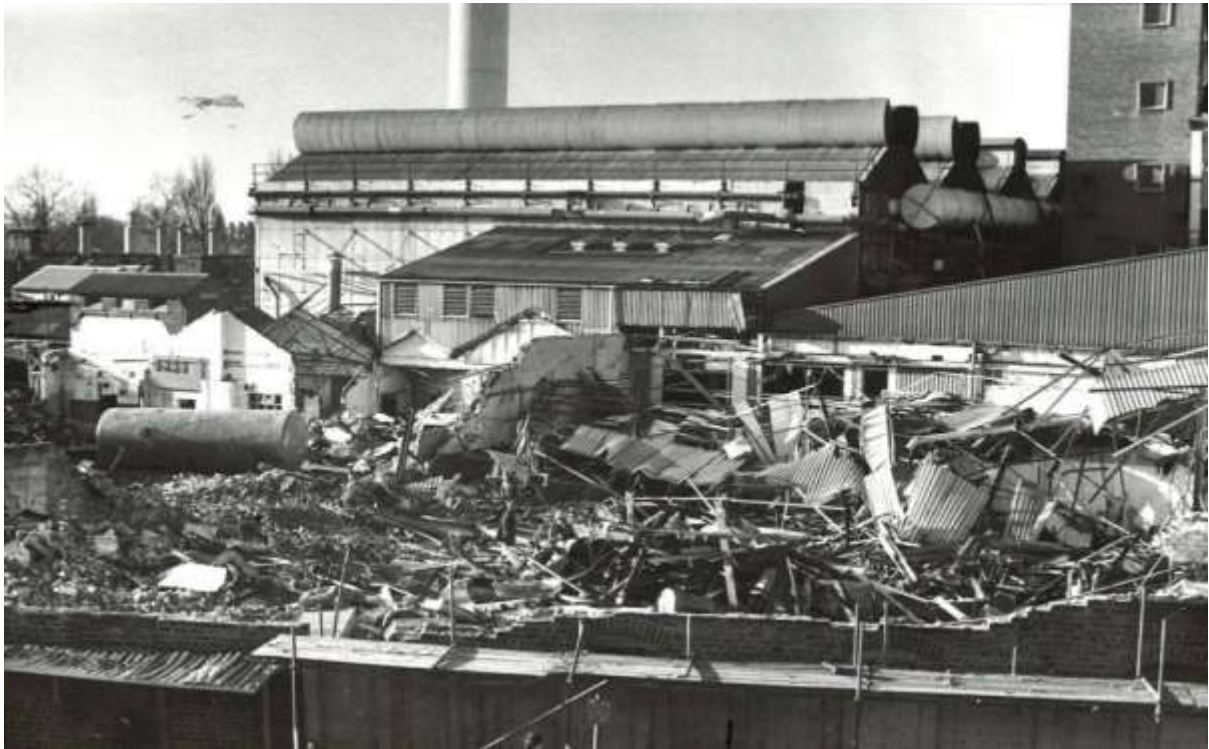
Demolition in progress. Image: York Press
