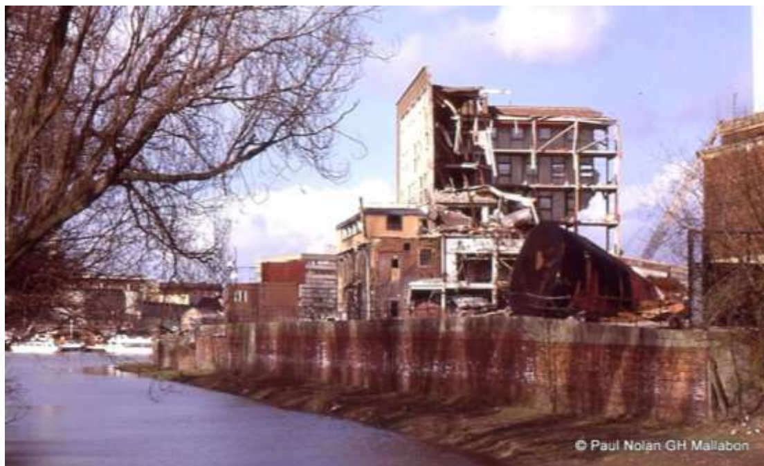
The Glassworks during demolition c.1984. Image Paul Nolan
