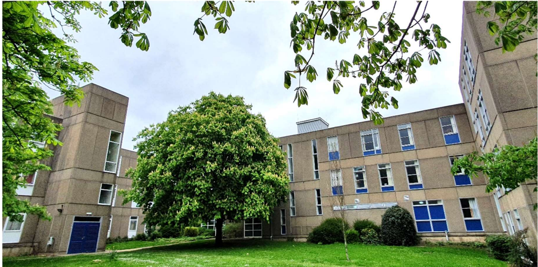
View of Derwent Block P on the left (with window replacements) and the originals on the right.
