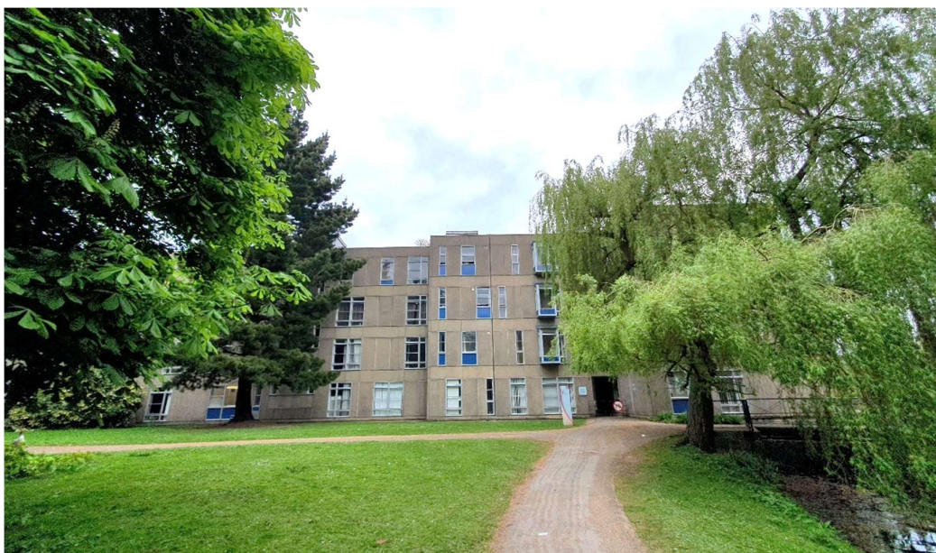
View looking towards the entrance of Derwent College
