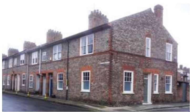
The small window over the passageway in Farndale Street (Pictured left) shows where the front bedroom has been divided to create a bathroom. The adjoining house will have its bathroom over the passage at the back. The same applies to Levisham Street (pictured right) where the soil and vent pipes can be seen above the passage on two houses
