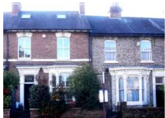
Houses in Grange Crescent on Fulford Road. The windows and doorways are very similar but bricks and other details are different. Woodwork around the windows and doors has elaborate carving, similar to those on the Villas.
