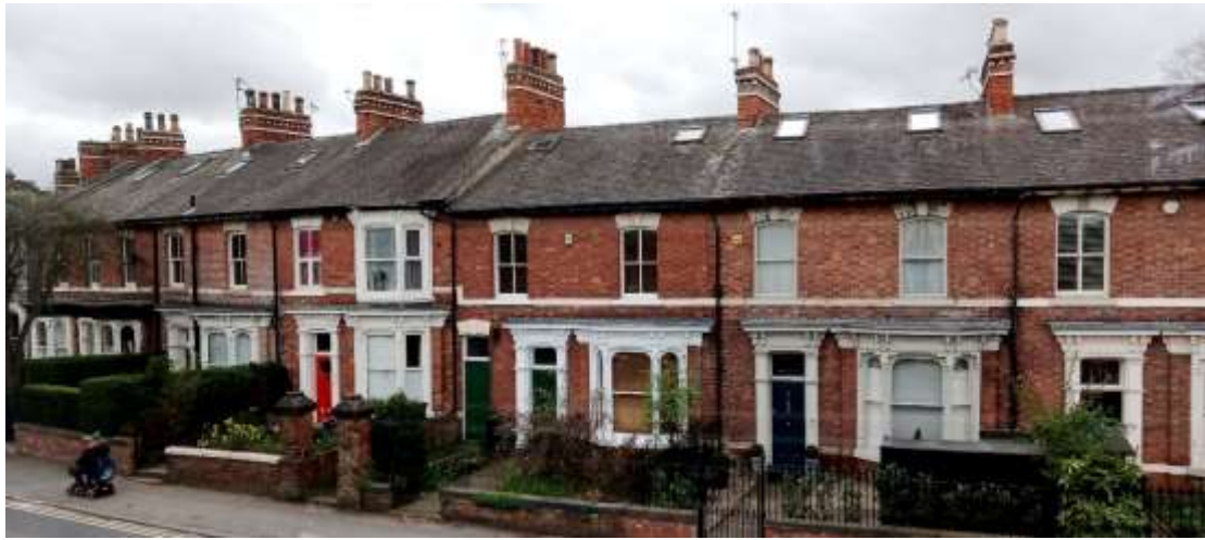
Houses in Grange Crescent, Fulford Road, have ornate wood mouldings to the doors and windows. The house with the red door has a matching bay window to the front bedroom. It looks somewhat like a later addition, but it can be seen on a photograph of c.1911, so it may be original.
