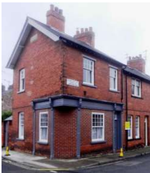
Former shops in Hartoft Street: No 1
