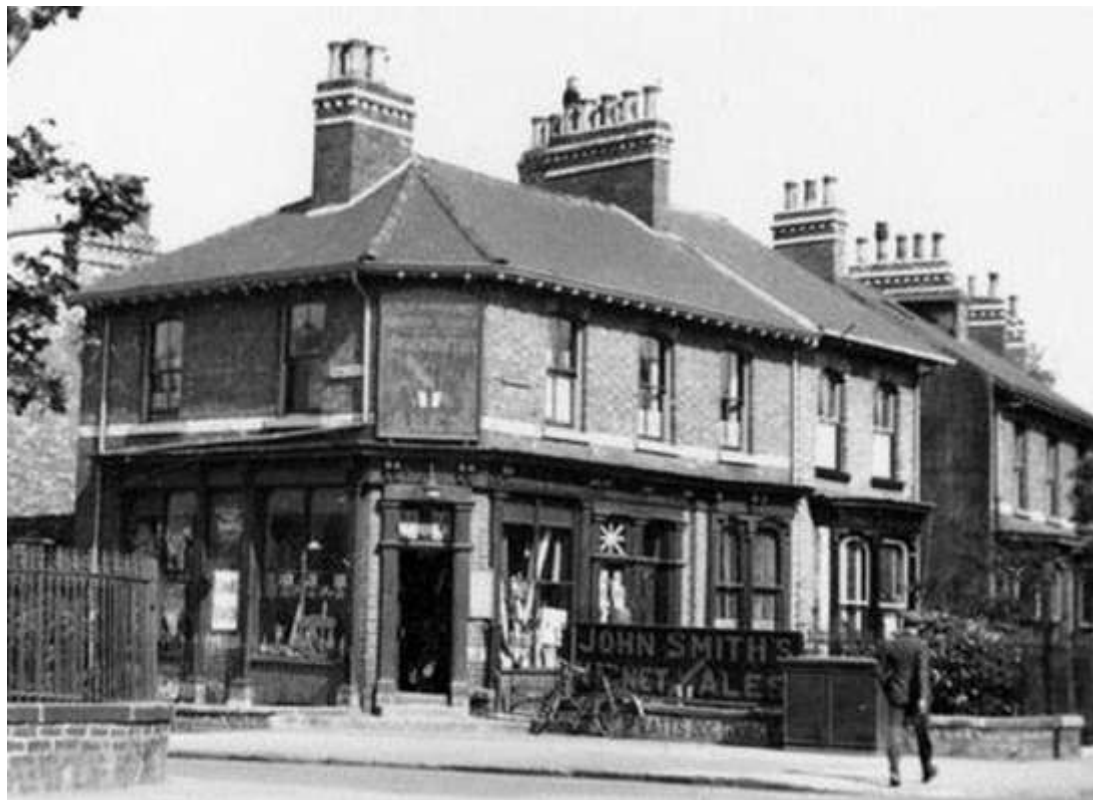
'Cooper's Corner' shop on the corner of Grange Street pictured in 1935.
