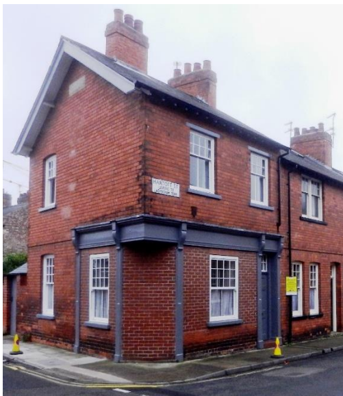
Former shops in Hartoft Street: No 1
