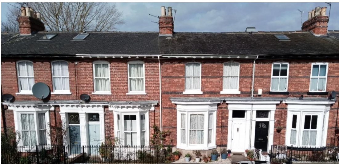
Houses in Grange Street (north side) with square front doorways. Note the small changes of style
