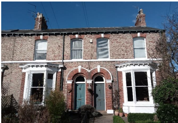
Houses in New Walk Terrace with arched front doorways, built in 1876
