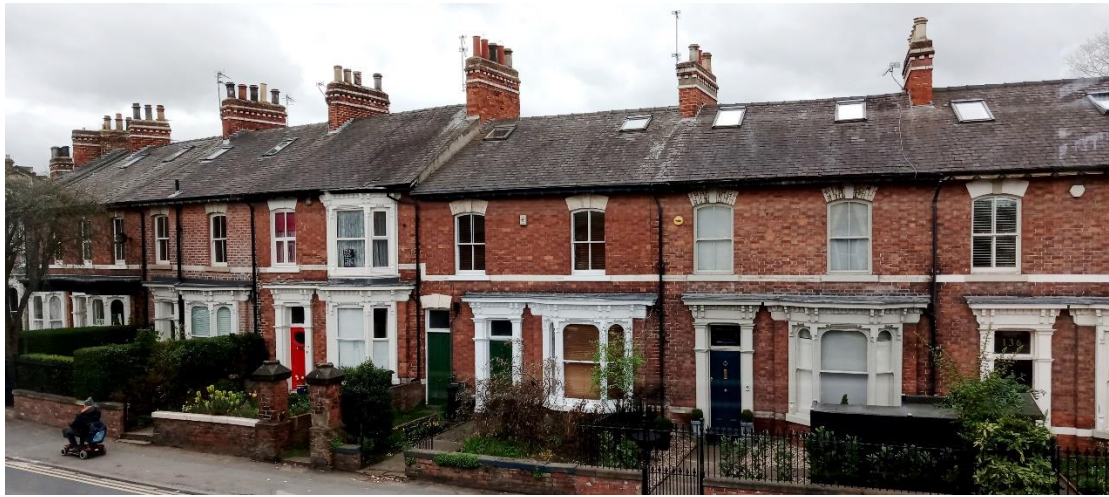
Houses in Grange Crescent, Fulford Road, have ornate wood mouldings to the doors and windows. The house with the red door has a matching bay window to the front bedroom. It looks somewhat like a later addition, but it can be seen on a photograph of c.1911, so it may be original.
