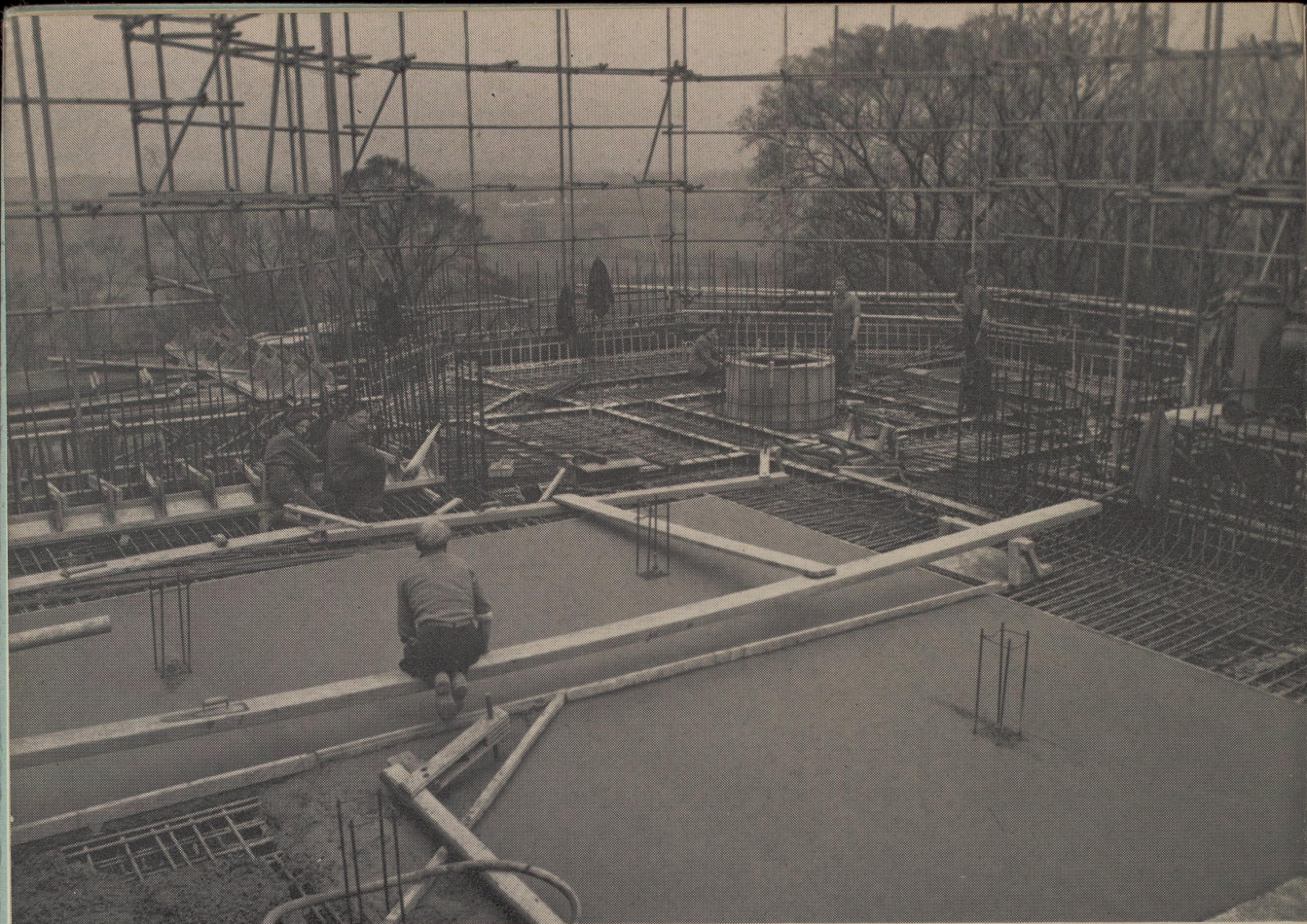
Concreting tank floor, South West corner.
